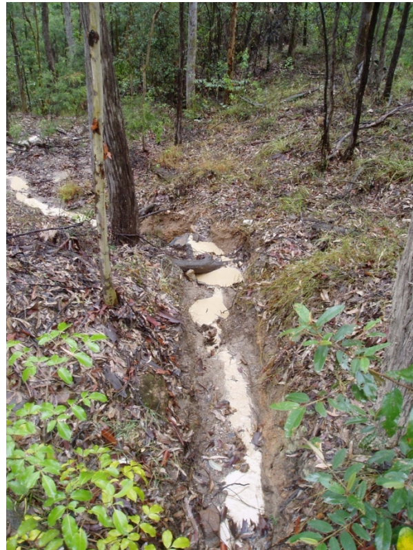
Fig. 7. Gully below a relief pipe conveying sediment laden water and exhibiting full stream connectivity
