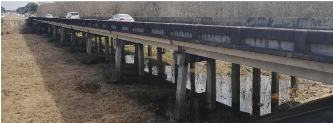
Figure 2. Side view of the bridge.
